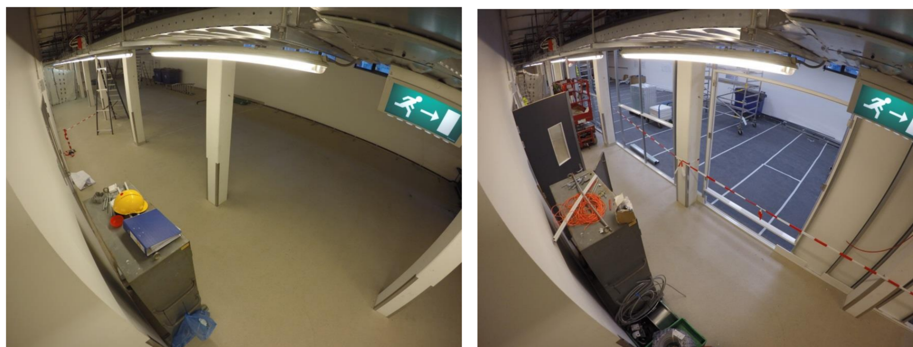
Figure 2: clean room area under construction
